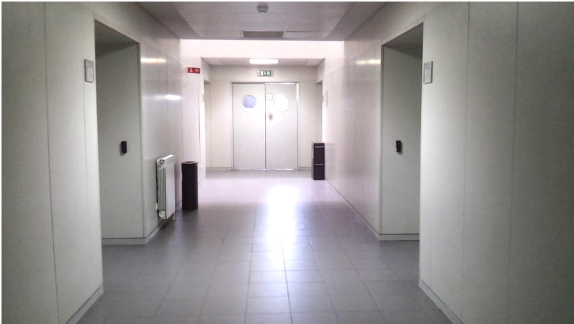
Figure 4.5: Example of two recessed doors as seen by the drone
