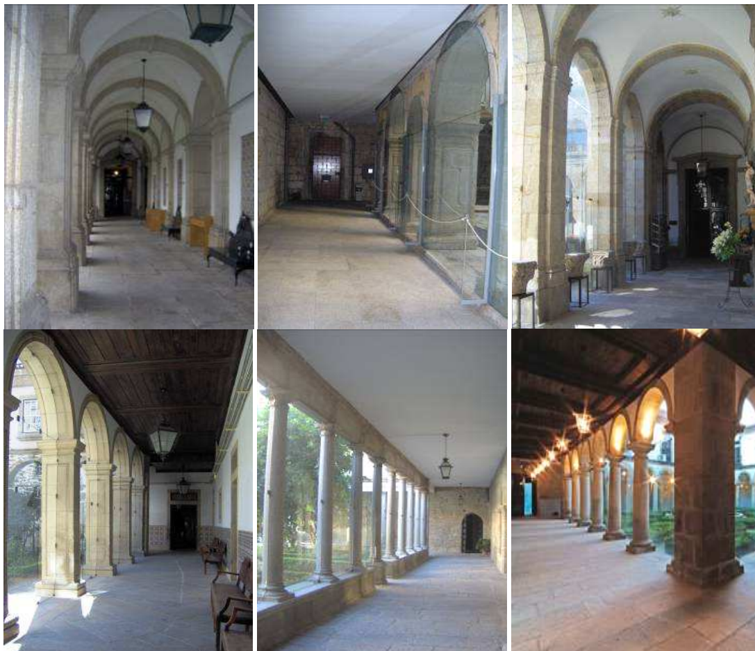
Fig. 1 to 6 The six studied cloisters with the rehabilitated galleries: openings between galleries and central yard closed with glass (top left to bottom right: BP, PSP, SB, ESE, SF, and CA) [3].
