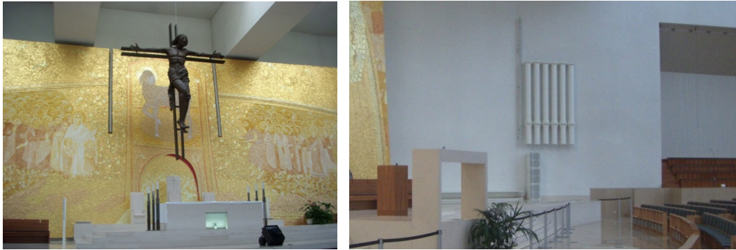
Figures 10 and 11 – Suspended loudspeakers (left) and loudspeakers and Wave Cannons for the organ (right).
