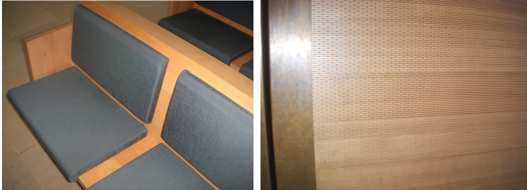
Figure 4 and 5 – Cushioned pews (left) and perforated panels (right).
