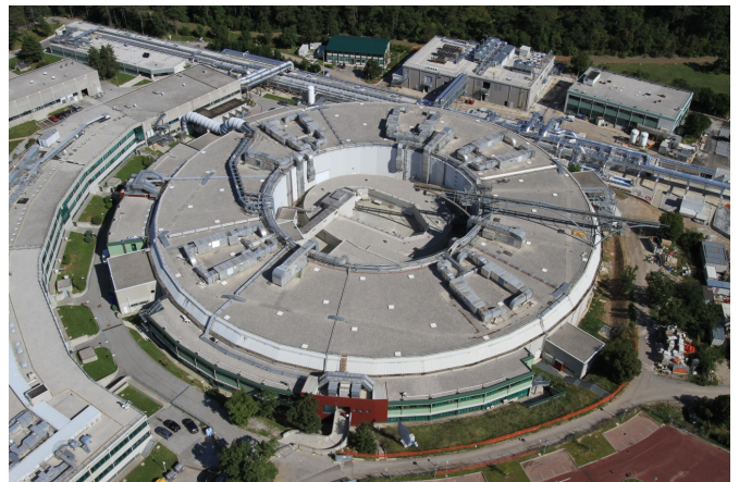
Fig. 4. - Aerial view of the building hosting Elettra Storage Ring (SR).
