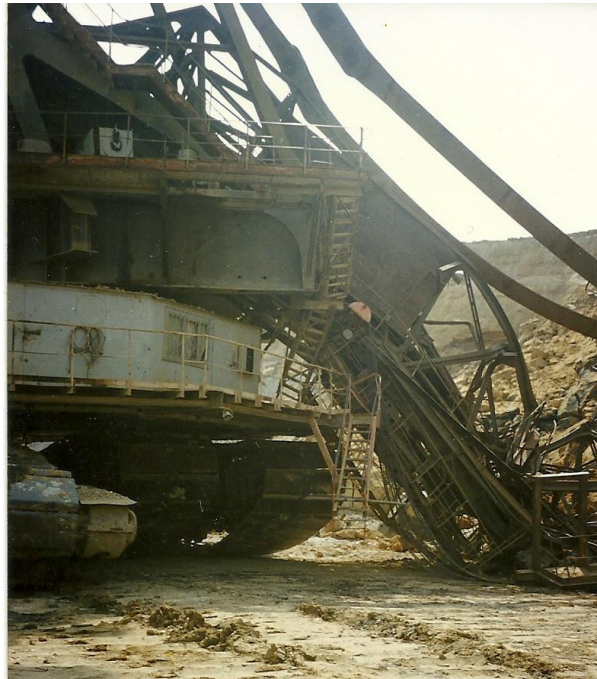
Figure 1 – The collapse of a bucket wheel excavator ESRC 470
