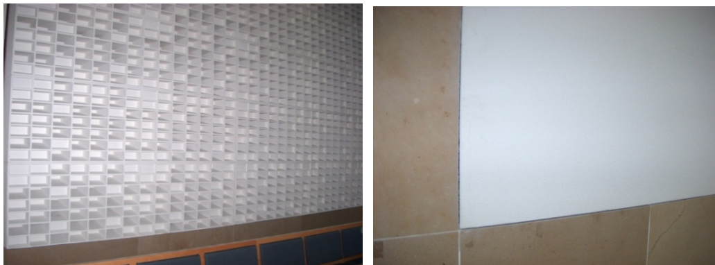
Figures 8 and 9 – Diffusers (on the congregation rear wall) (left) and wall with absorptive Akustaplan (white on photo at right).
