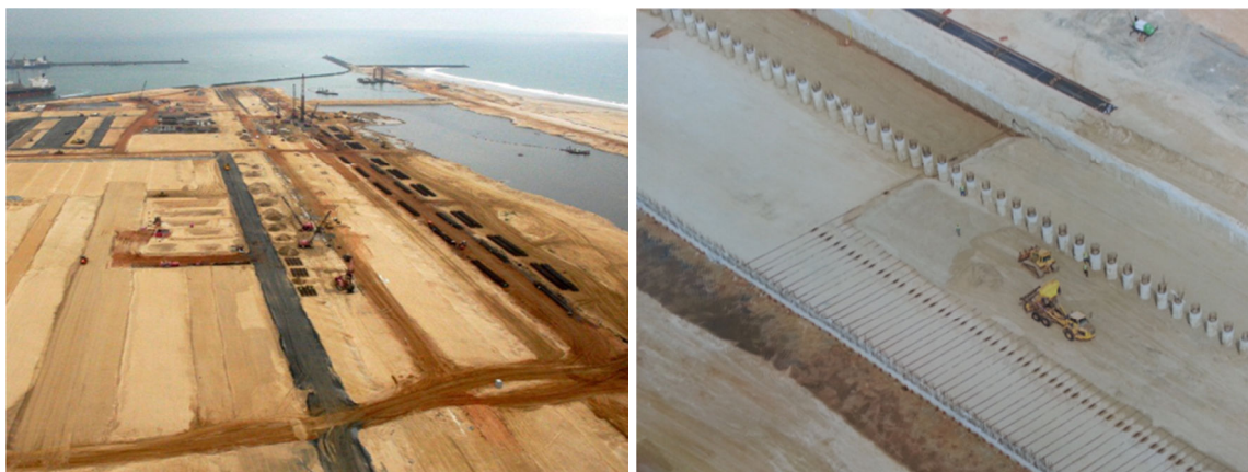
Fig. 2 - Global view of the works
