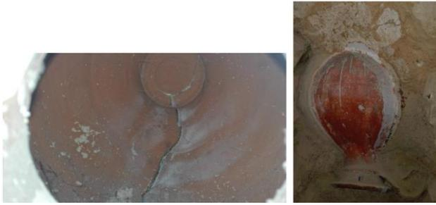
**Figure 3.** Acoustic vases: on the left the interior of one of the vases; on the right one of the uncovered vase [8].
