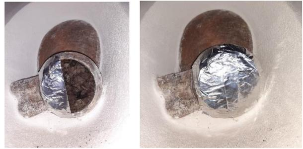
**Figure 5.** Occlusion of acoustic vases, using "lids" of black cork agglomerated and externally covered with aluminum foil.
