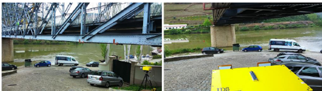
Fig. 9 - Positioning of radar IBIS-FS for SHM along longitudinal direction from (Alves, 2016).
