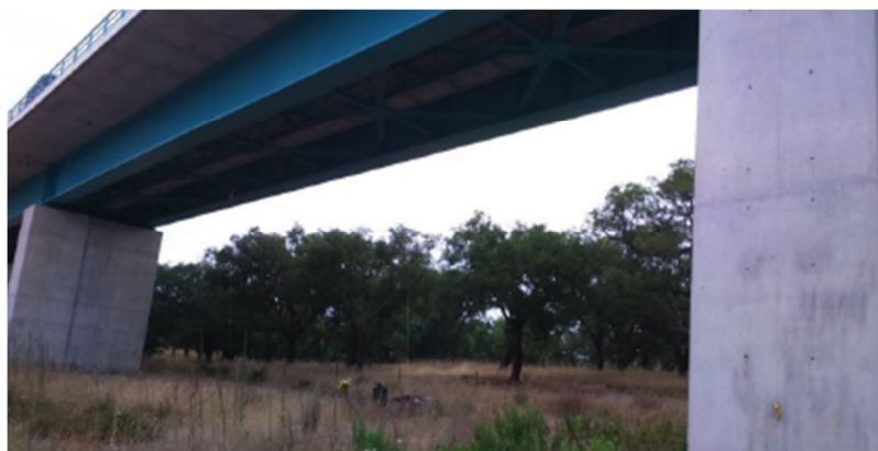
Fig. 16. Simply supported viaduct of Alcacer bridge under SHM from (Alves,2016)
