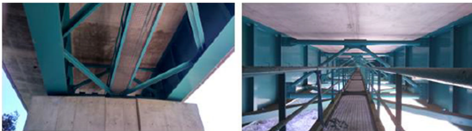
Fig. 17 - Structural metallic elements (bracing, diaphragms and walkaway) of the viaduct stretch under SHM from (Alves,2016)
