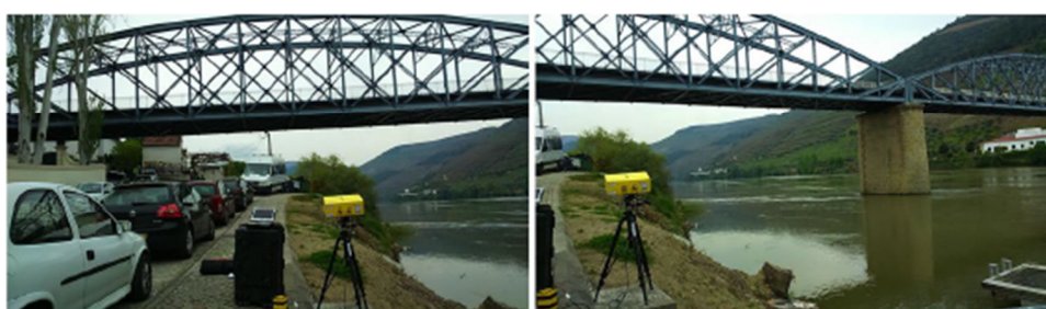
Fig. 12 - Positioning of radar IBIS-FS for SHM along transversal direction from (Alves, 2016).
