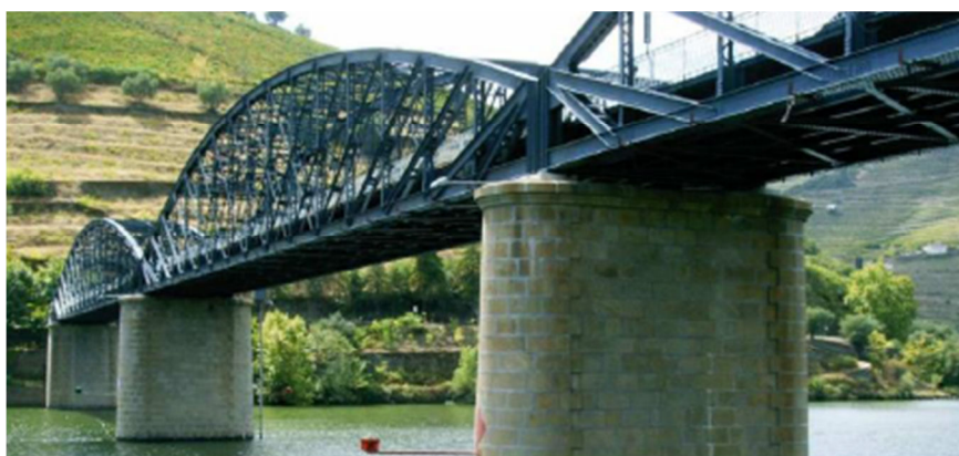
Fig. 7 - Pinhão Bridge from (Alves, 2016)
