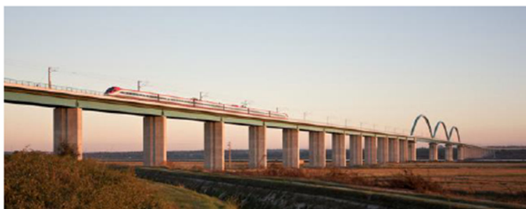
Fig. 15 -General view of Alcacer-do-Sal bridge from (Reis, 2010).
