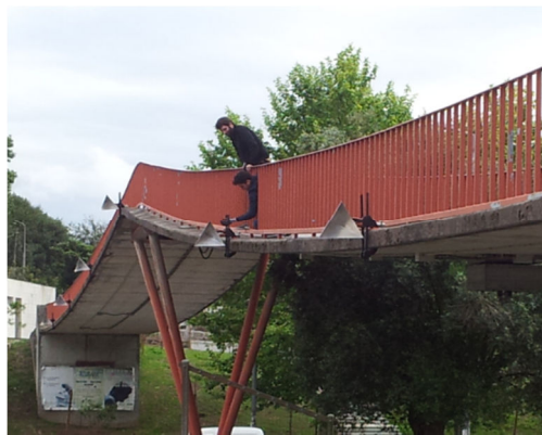
Fig. 3 - Installation of the reflective cones (Silva, 2015)
